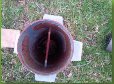
Bolt attachment through drop tube allows moisture to enter, Note rust!
